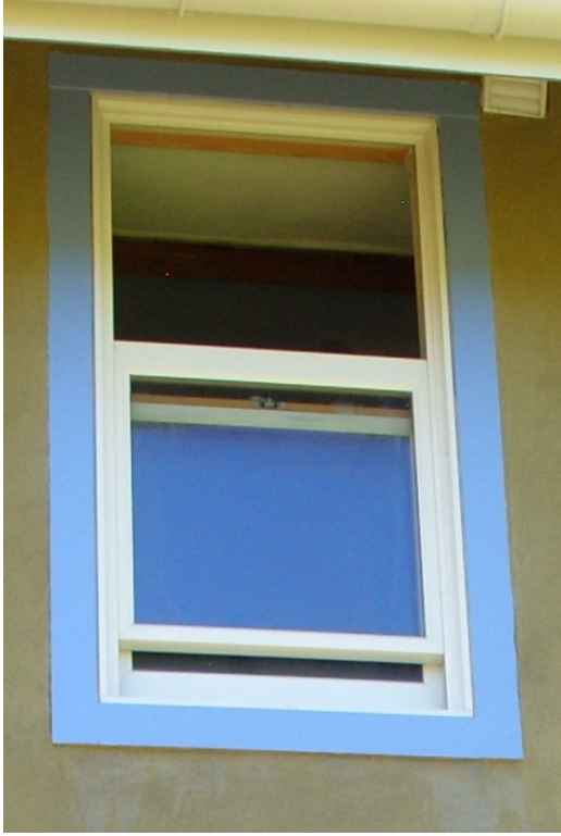
Figure 26 Double hung window at ELC.
