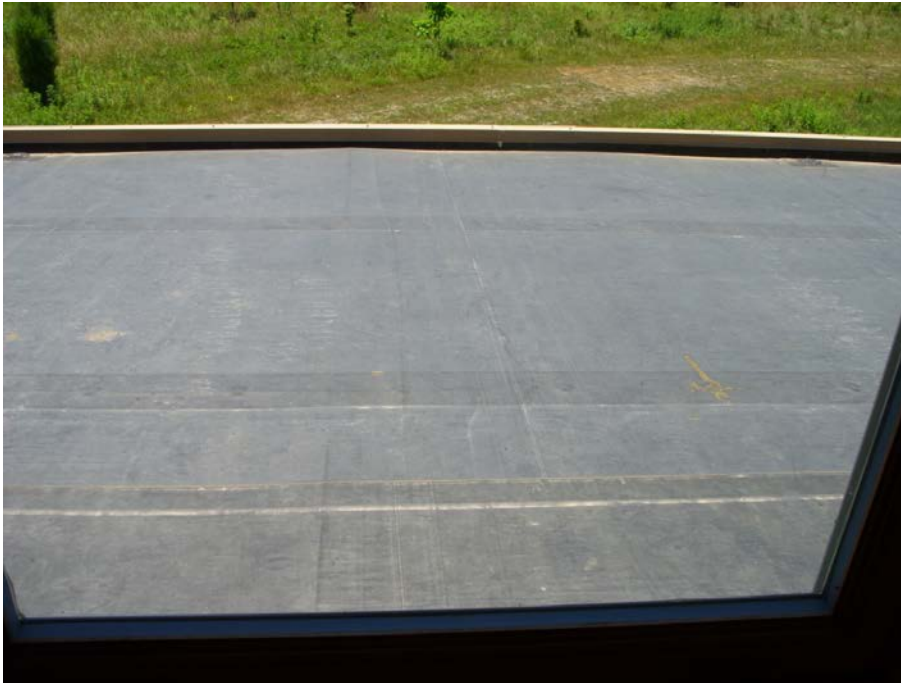
Figure 18 Waterproof membrane for green roof.
