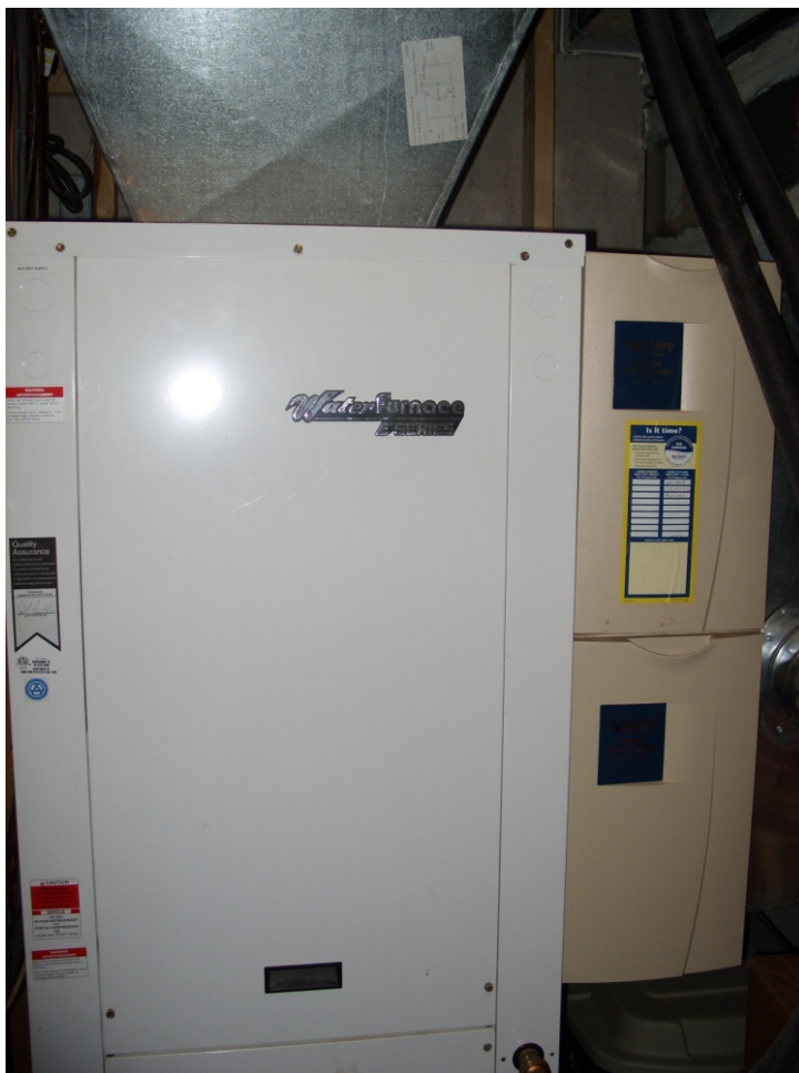
Figure 24 Geothermal system at CC home.
