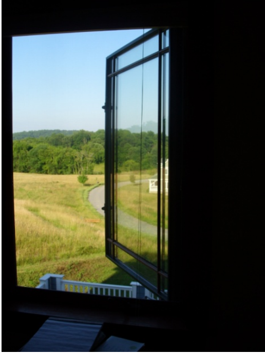
Figure 25 Casement window at CC.
