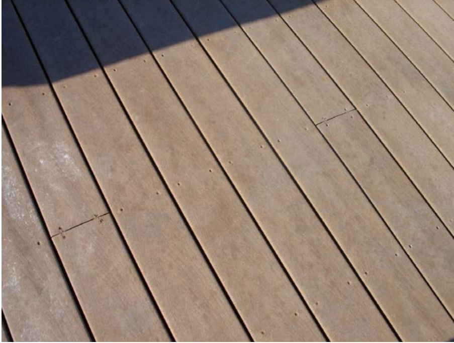
Figure 27 Trex decking from home at CC.
