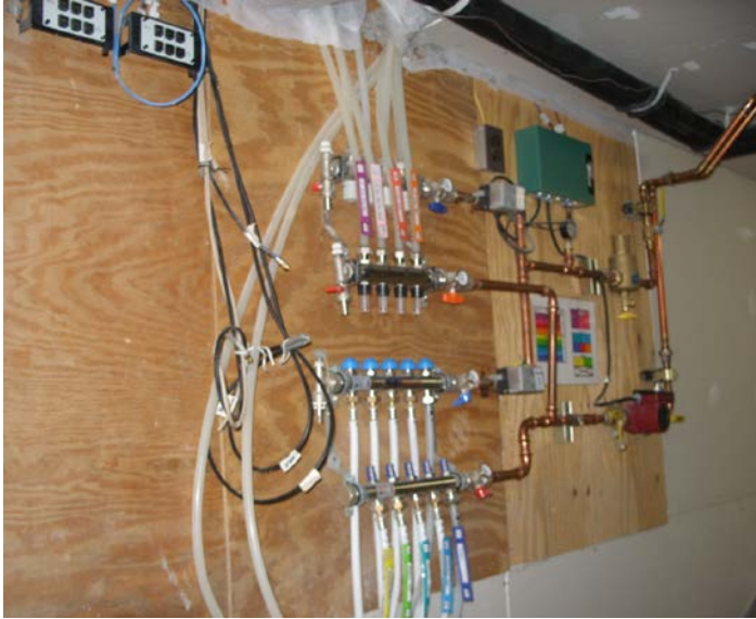
Figure 21 Plumbing for radiant flooring.
